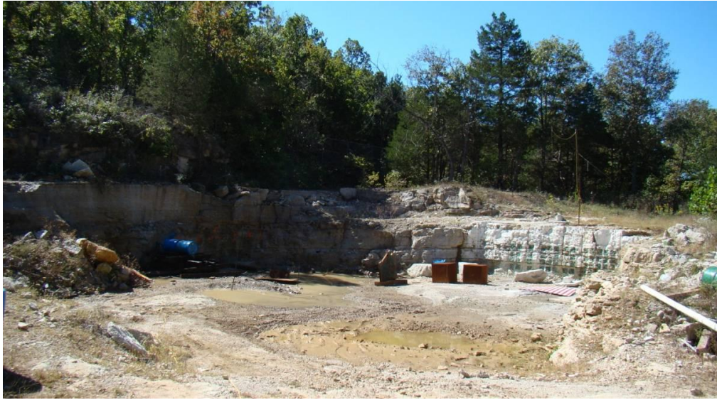
Figure 4.1 Above Ground Testing Facility
